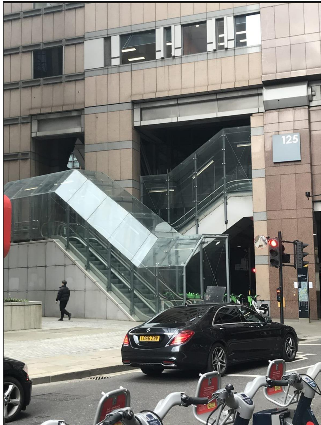
Existing Site Photos Wood Street (south side)
