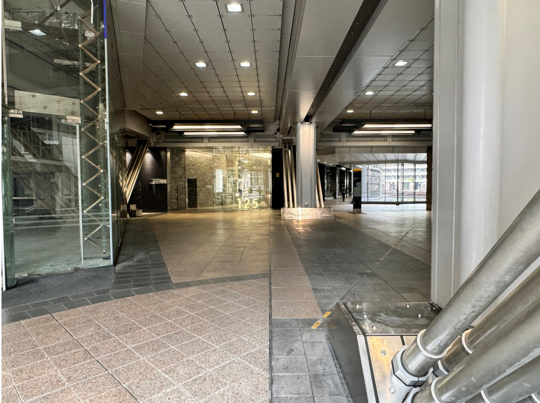
Existing Site Photos looking north across Alban Highwalk
